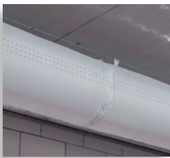
MICRO-PERFORATED FABRIC DUCT high induction duct PG. 88
