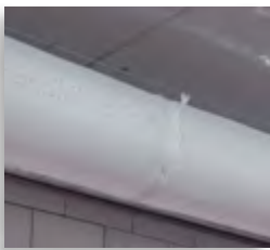
MICRO-PERFORATED FABRIC CHANNEL high induction channel PG. 88
